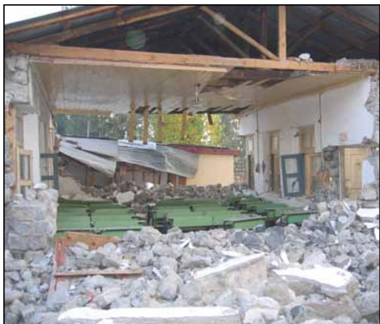
**Figure 2.28** Out-of-plane collapse of two parallel walls, NWFP Pakistan (photo: SDC)
