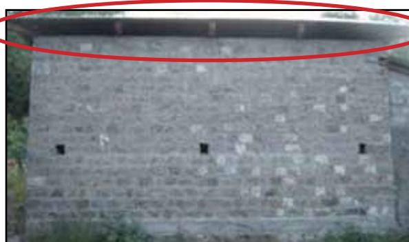
**Figure 2.10** A stone masonry building in Muzzaffarabad was undamaged in the 2005 Kashmir, Pakistan, earthquake; this was attributed to the presence of an RC band at the eaves level (photo: J. Bothara)
