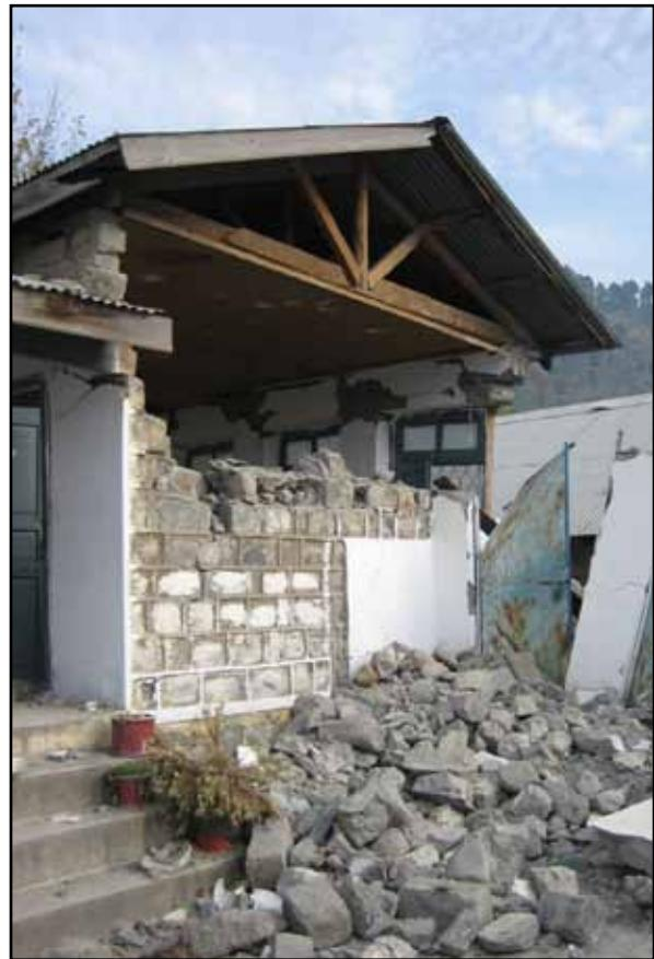
**Figure 1.13** Timber truss roof structure in the area affected by the 2005 Kashmir earthquake in Pakistan (source: M. Tomazevic 1999)
