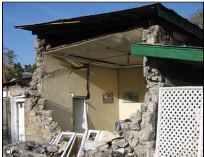
**Figure 2.30** Out-of-plane collapse of stone masonry walls in buildings with flexible roofs and inadequate wall-to-roof connections:
