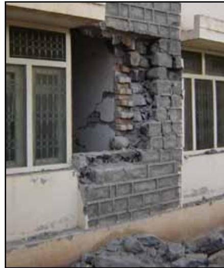
**Figure 2.38** Vertical cracking at a wall intersection in the 2005 Kashmir, Pakistan, earthquake due to absence of connection between the intersecting walls, a stone masonry and a brick-masonry wall (source: Bothara and Hiçyilmaz 2008)
