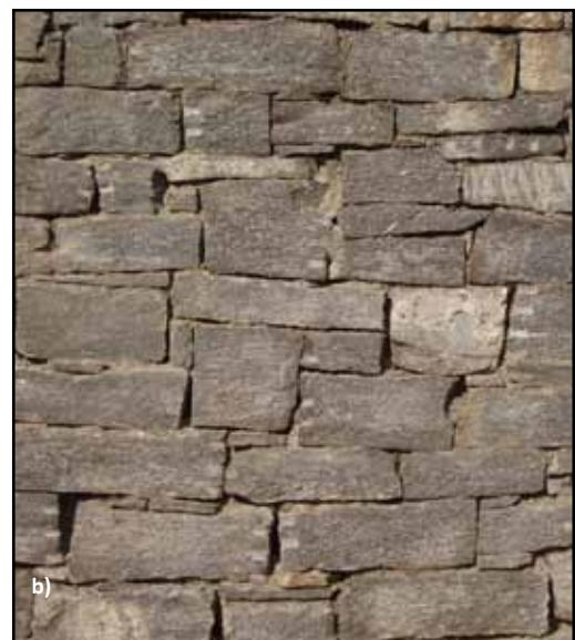
**Figure 1.32** Dressed stone masonry construction in Southern Switzerland: a) a typical building in Giornico, and b) a detail of the exterior (photos: T. Schacher)
