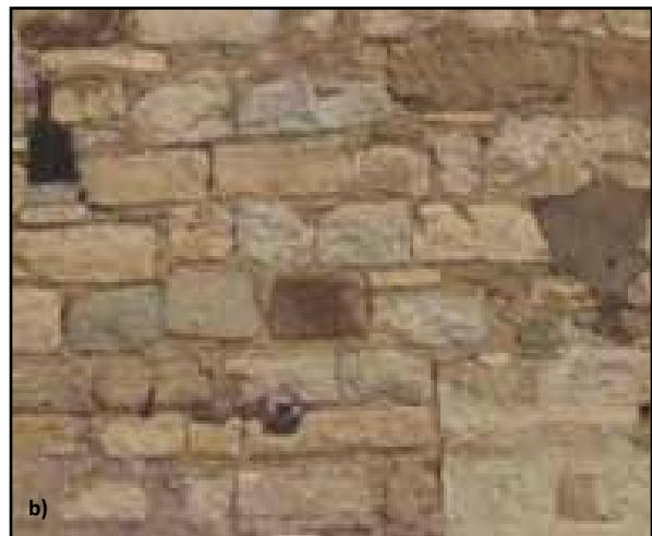
**Figure 1.31** Dressed stone masonry: a) an isometric view of a typical wall, and b) an exterior of a wall in Umbria, Italy (source: Maffei et al. 2006)
