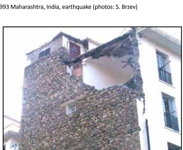
**Figure 2.25** Out-of-plane collapse at the top floor of a stone masonry building in the 2003 Boumerdes earthquake in Algeria (photo: M. Farsi)
