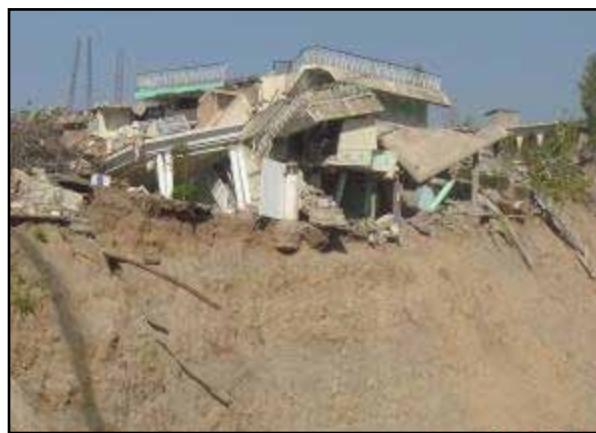
Figure 3.3 A building damaged by a landslide in the 2005 Kashmir, Pakistan, earthquake (source: Bothara and Hicilmaz 2008)
