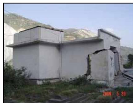
**Figure 2.39** Soil spreading in the 2005 Kashmir, Pakistan, earthquake - note wide cracks in the walls (source: Bothara and Hiçyilmaz 2008)
