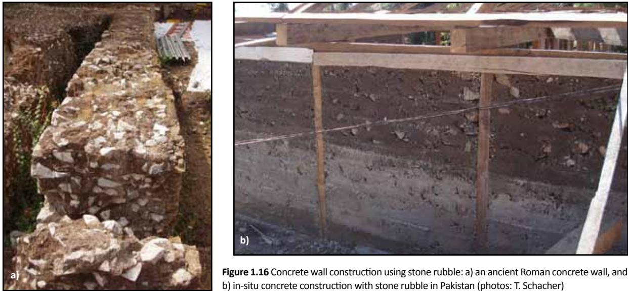
**Figure 1.16** Concrete wall construction using stone rubble: a) an ancient Roman concrete wall, and b) in-situ concrete construction with stone rubble in Pakistan (photos: T. Schacher)
