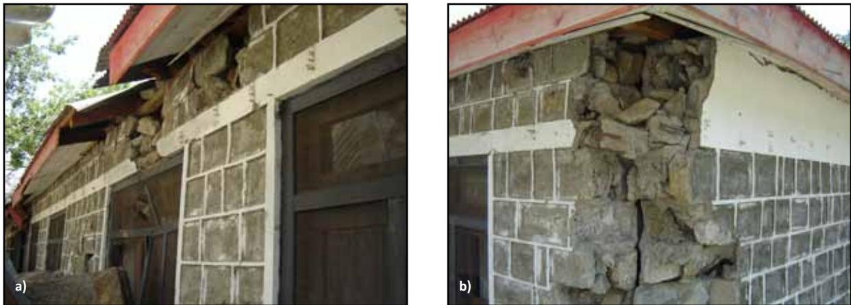
**Figure 2.11** A stone masonry building with an RC lintel band that survived the 2005 Kashmir earthquake in Pakistan: a) the building suffered only moderate damage in the top portion, and b) separation at the wall intersection took place in spite of the band (note inadequate anchorage of the band reinforcement) (photos: Builders Without Borders)
