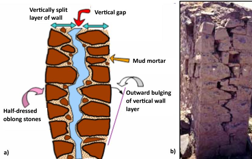
**Figure 2.20** Delamination of stone masonry walls: a) delamination in progress (source: Murty 2005), and b) delamination of wall wythes due to the 1993 Maharashtra, India, earthquake (photo: S. Brzev)
