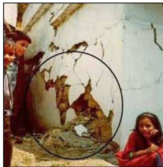
**Figure 2.35** Localized wall failure caused by irregular stones (source: WHE Report 74)
