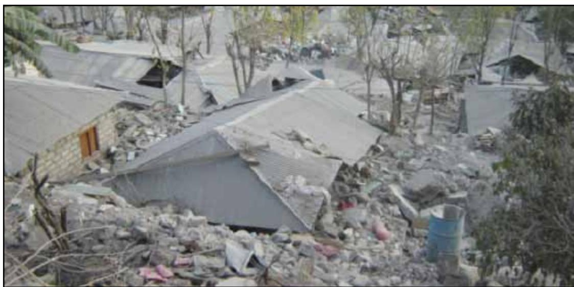
**Figure 2.17** Collapse of stone masonry buildings with hipped roofs in the 2005 Kashmir, Pakistan, earthquake (source: Bothara and Hicyilmaz 2008)
