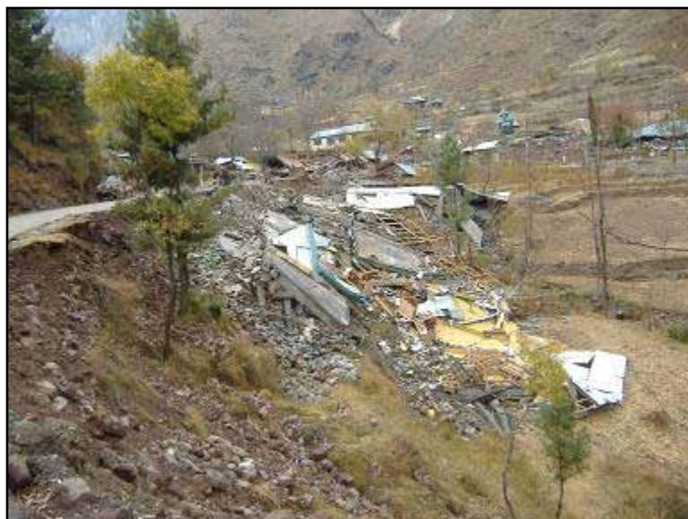
**Figure 3.1** A collapsed building on a steep slope after the 2005 Kashmir earthquake, Pakistan (source: Bothara and Hicyilmaz 2008)
