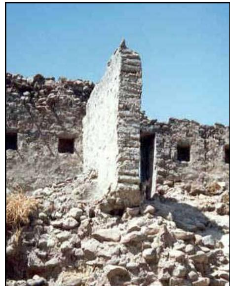
**Figure 1.18** A wall without foundations in the area affected by the 1993 Maharashtra, India, earthquake (photo: S. Brzev)
