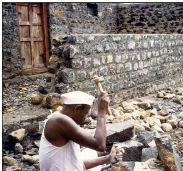
Stone masonry walls can be classified into three types: uncoursed random rubble stone, uncoursed semi-dressed stone, and dressed stone. This classification is made based on the type of stone, extent of shaping, and the layout. In all these wall construction types, common deficiencies include: lean cement mortar, the use of soil or very fine sand mixed with sea sand, and the absence of curing.
