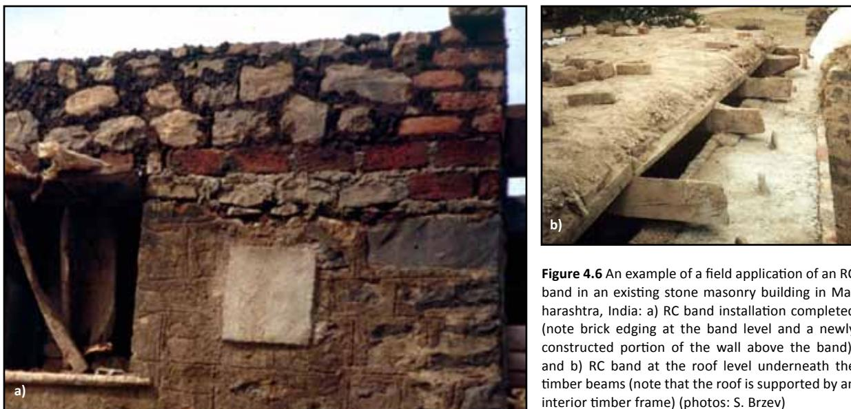
**Figure 4.6** An example of a field application of an RC band in an existing stone masonry building in Maharashtra, India: a) RC band installation completed (note brick edging at the band level and a newly constructed portion of the wall above the band), and b) RC band at the roof level underneath the timber beams (note that the roof is supported by an interior timber frame) (photos: S. Brzev)
