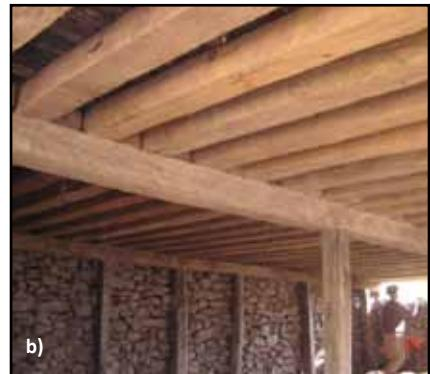
Figure 1.7 Dual gravity load-bearing system: a) a typical stone masonry building with exterior stone masonry walls and an interior timber frame in Maharashtra, India (source: GOM 1998), and b) a stone masonry building with dual system under construction in Pakistan (source: Bothara and Hiçyılmaz 2008)
