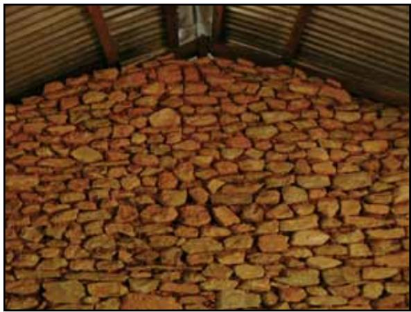
**Figure 2.31** A tall gable wall in Nepal that is at risk due to the absence of a wall-to-roof connection (photo: Smart Shelter Foundation)
