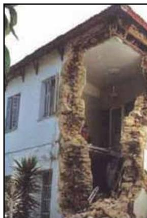
**Figure 2.8** Disintegration of stone masonry walls in Greece (source: WHE Report 16)
