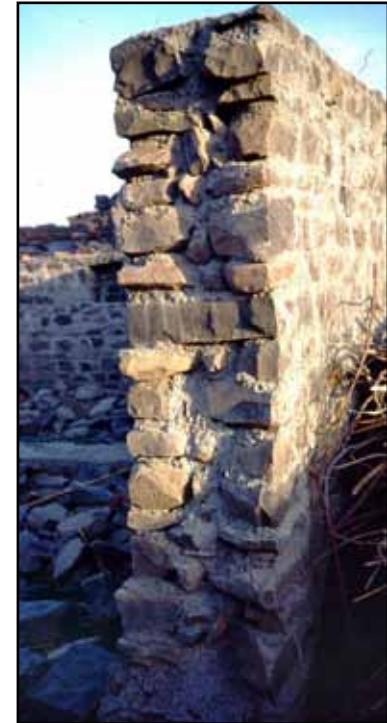
Through-stones extending over the full wall thickness must be used every 600 mm in height and at a 1.2 m maximum spacing along the length (Figure 3.29). Constructing walls in lifts not exceeding 600 mm can facilitate the installation of through-stones.
