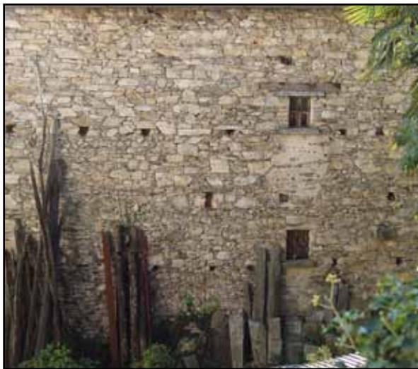
**Figure 1.26** Uncoursed semi-dressed stone masonry wall in Southern Switzerland (photo: T. Schacher)
