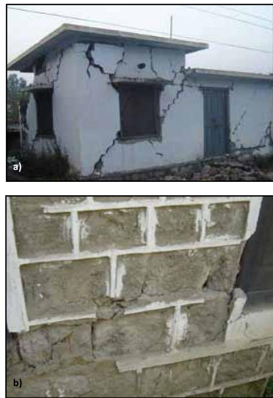
**Figure 2.34** Shear failure in stone masonry walls: a) shear cracks initiated at the corners of openings in the 2005 Kashmir, Pakistan, earthquake (Photo: Bothara and Hicyilmaz, 2008), and b) shear cracking in a stone masonry pier damaged by the same earthquake (photo: Builders Without Borders)
