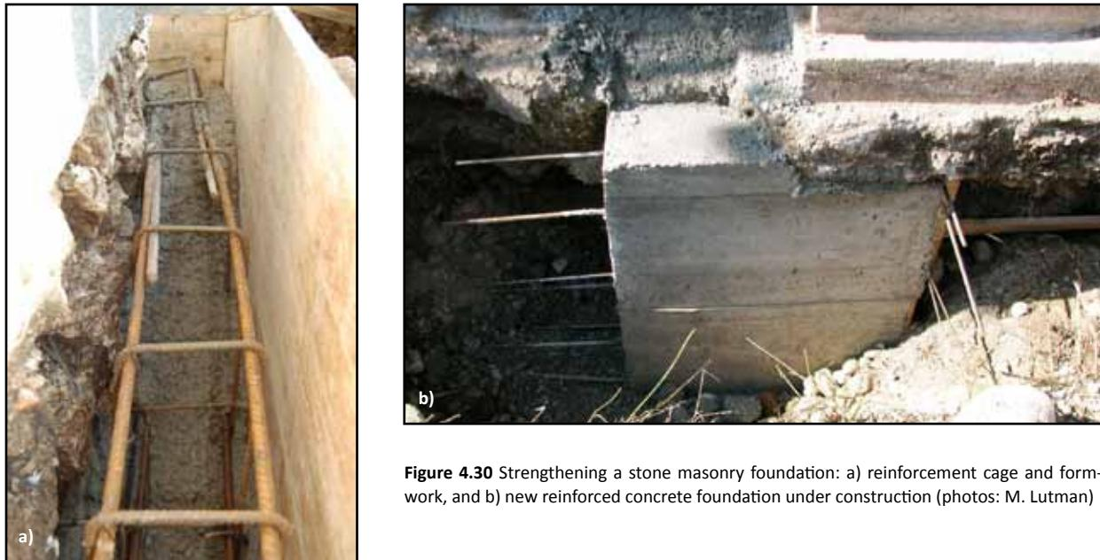
**Figure 4.30** Strengthening a stone masonry foundation: a) reinforcement cage and form-work, and b) new reinforced concrete foundation under construction (photos: M. Lutman)
