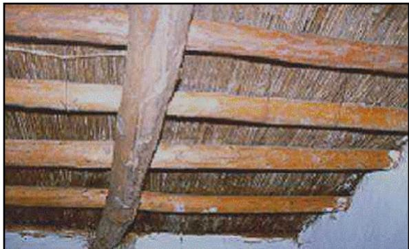
**Figure 1.11** A timber floor structure in Nepal (source: WHE Report 74)
