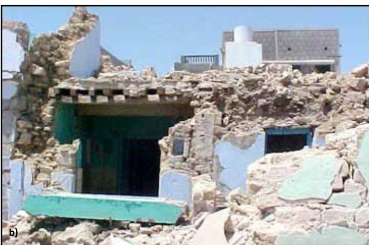
**Figure 2.14** Roof deficiencies in the area affected by the 2001 Bhuj, India, earthquake: a) discontinuous rafters over interior walls, and b) inadequate wall-to-floor connections caused the severe building damage (photos: C.V.R. Murty)
